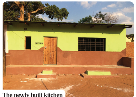
The newly built kitchen
