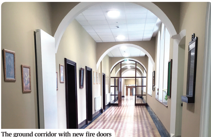
The ground corridor with new fire doors
