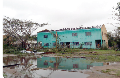
The roof of the hostel has been completely destroyed.
